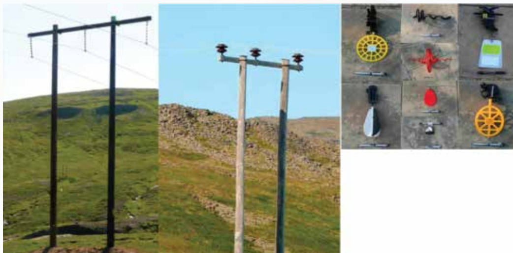
Figure 28: The threat from distribution lines. Left: A safe horizontal low voltage line, with 3 conductors suspended below cross-arm with long insulators. Centre: a low voltage line which is unsafe. Right: Bird Flight Diverters that can be fitted or retrofitted to avoid collisions.
